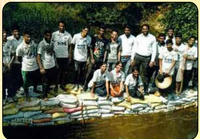
Construction of 'Check Dam' at Murnoli Village
